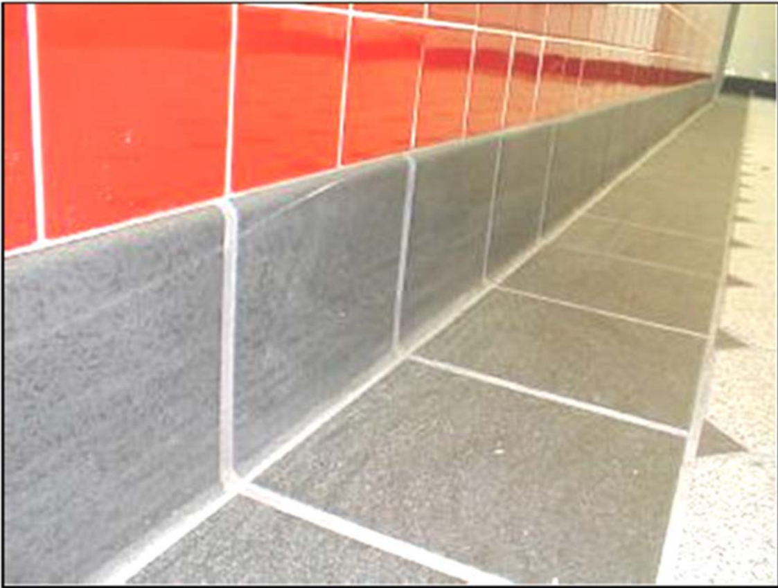
Figure 5. Ceramic Tiles with three eighths inch (3/8") Radius Cove
