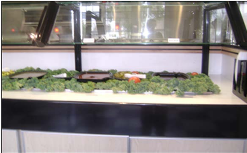
Figure 15. Sneeze Guards – Enclosed On End
